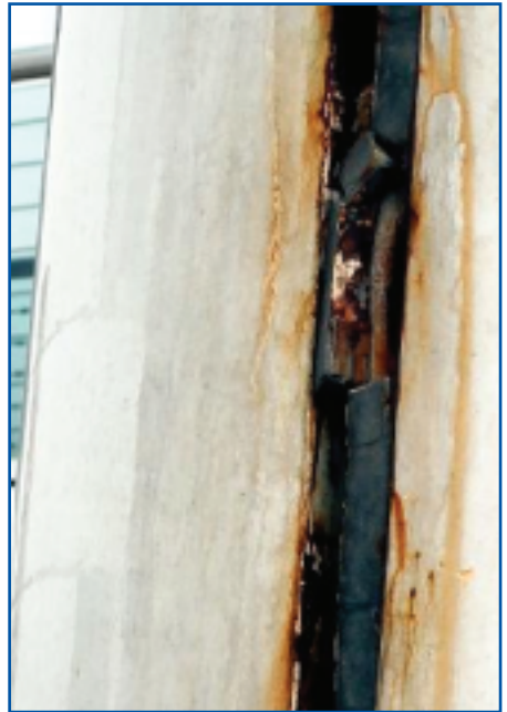
Figure 1. Corrosion to steelwork caused by water entering through a failed joint sealant.
